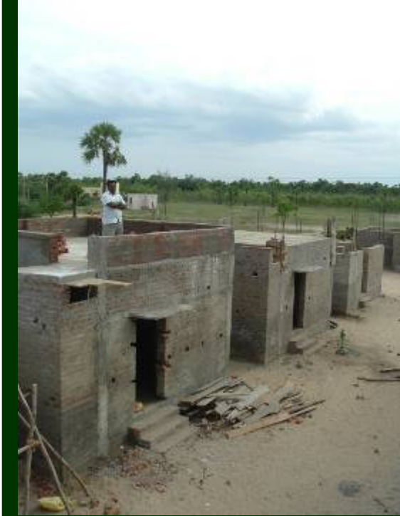
Over view of Roof Laid
