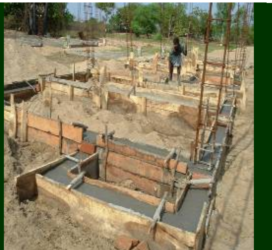
Processing Grade Beam
