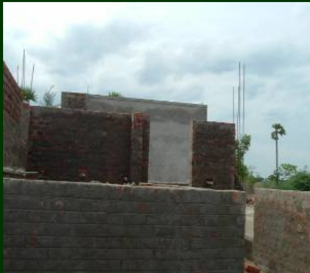
Above Basement Level
