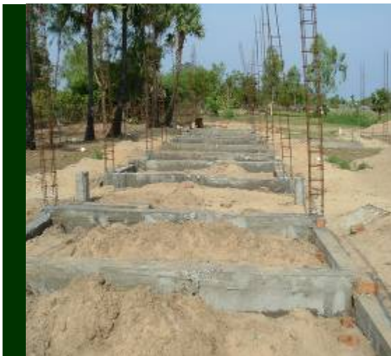
Grade Beam Laying
