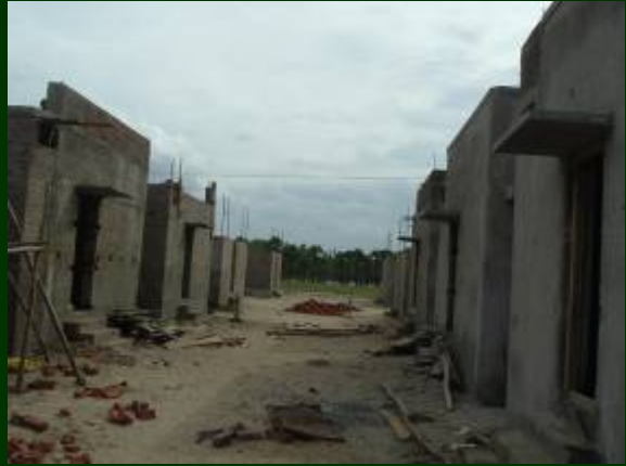
Over view of the row of Permanent Houses
