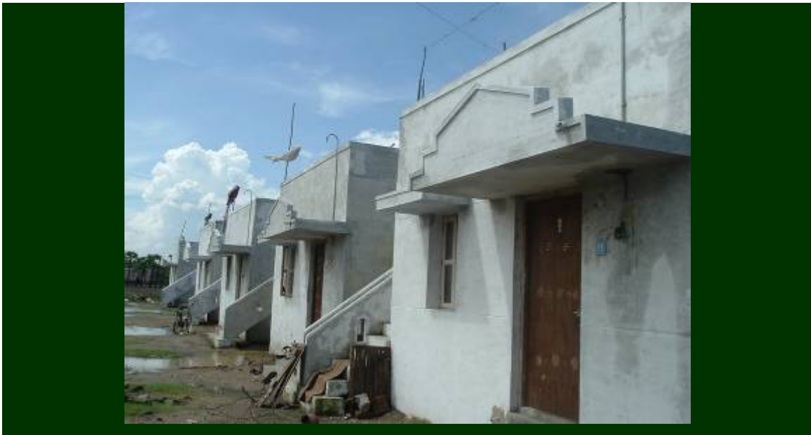
Over view of completed Permanent Houses
