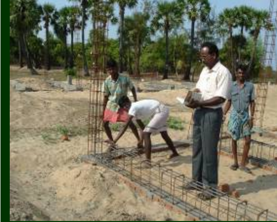
Grade Beam Steel Fabrication
