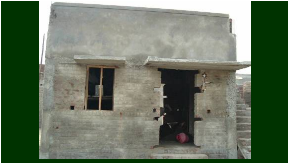
Plastering Work [Outer Plaster]
