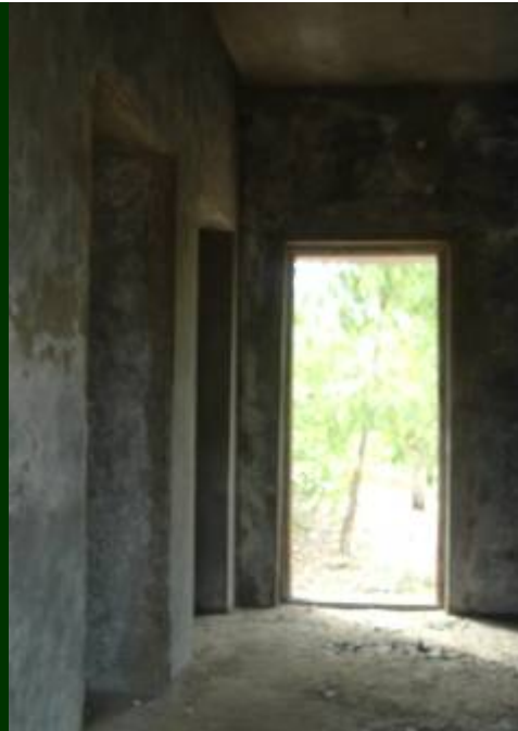
Roof Laid with Inner Plaster work completed
